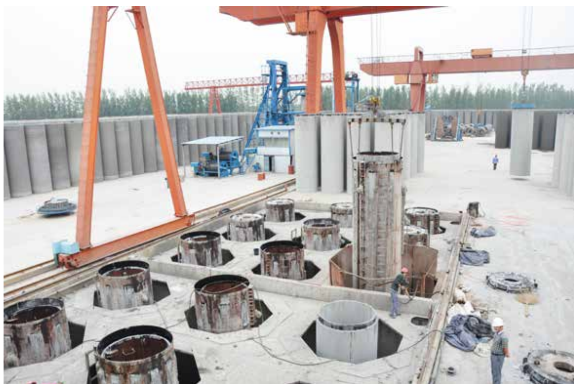
Vertical PCCP Molds Casting Platform
